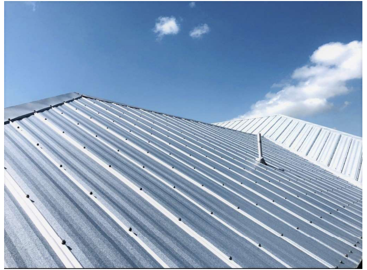
North side of roof
