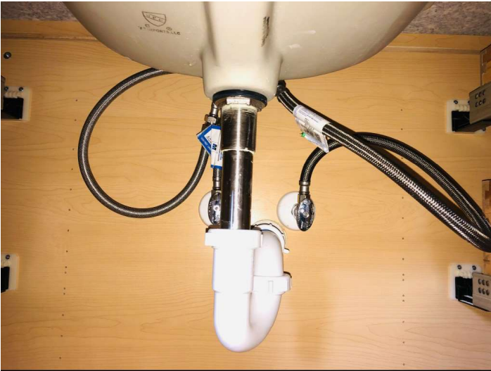
Bathroom #1 under sink 1
