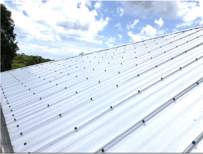
Back of roof
