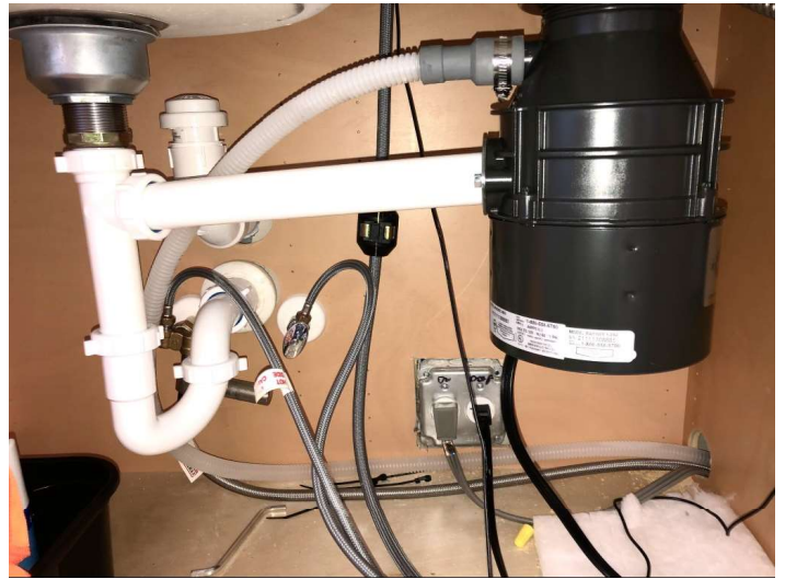
Under kitchen sink
