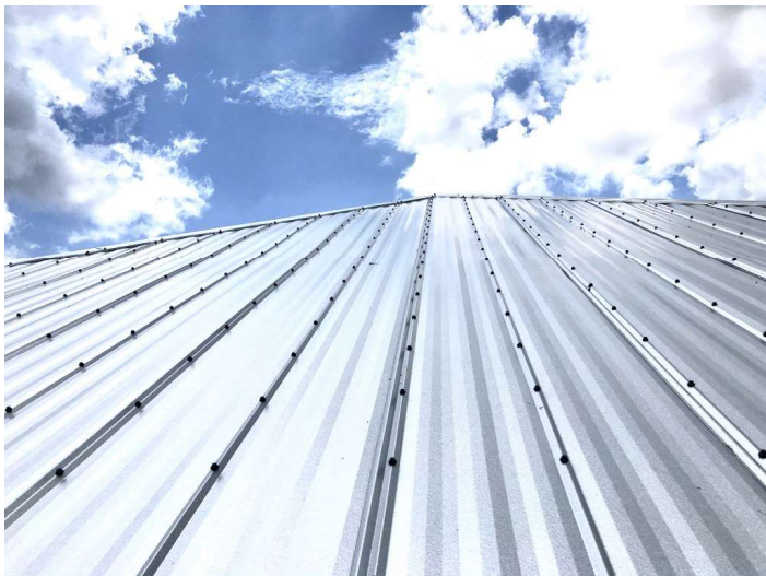
Front of roof
