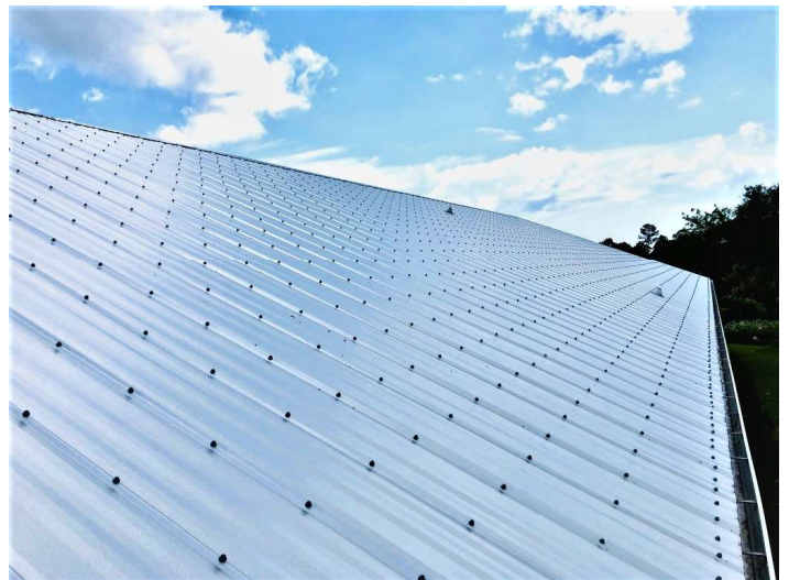
South side of roof
