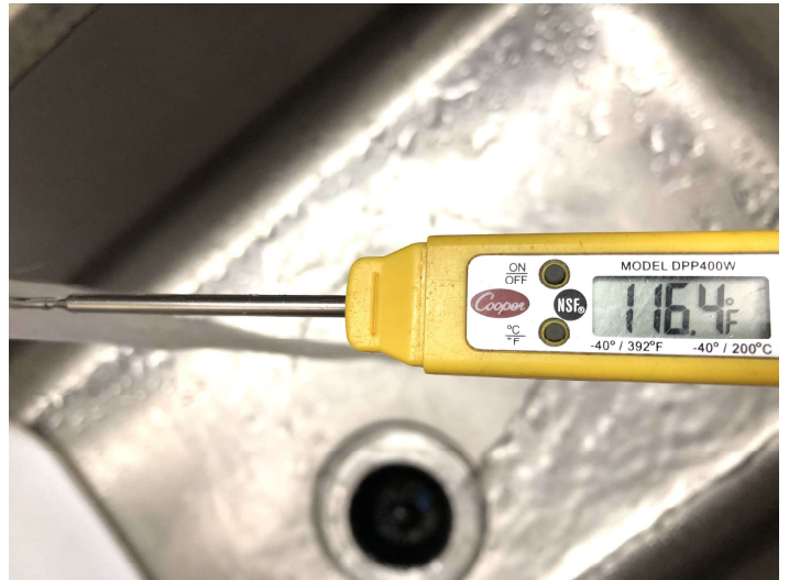
Hot water heater temperature 116.f (good)
