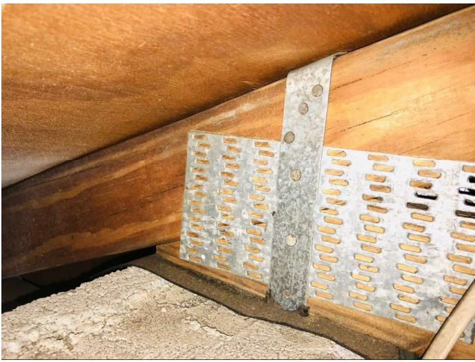
Single straps embedded in concrete nailed per code
