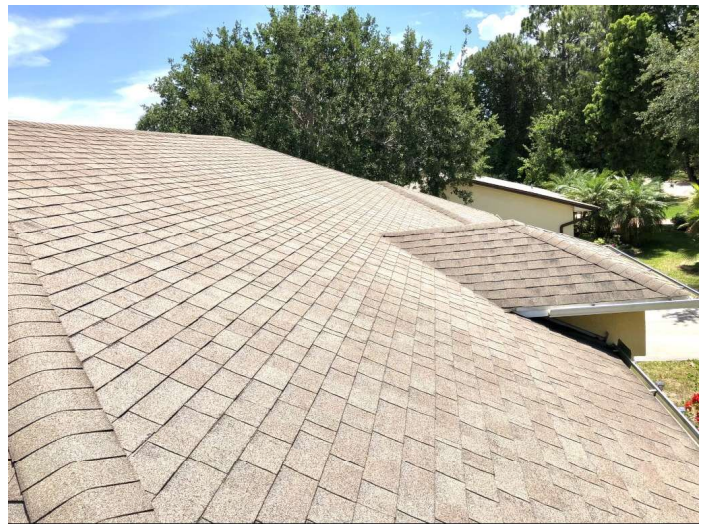
Southwest side of roof
