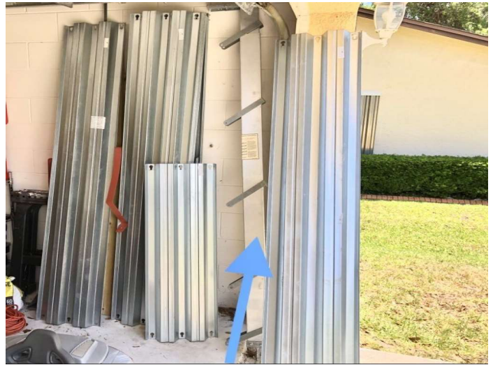
Shutter protection for all windows and doors - center beam (blue arrow)
