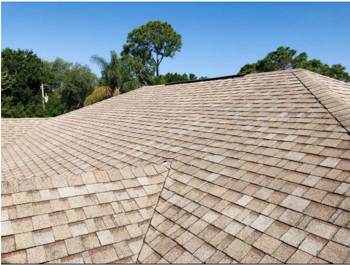
Northeast side of roof
