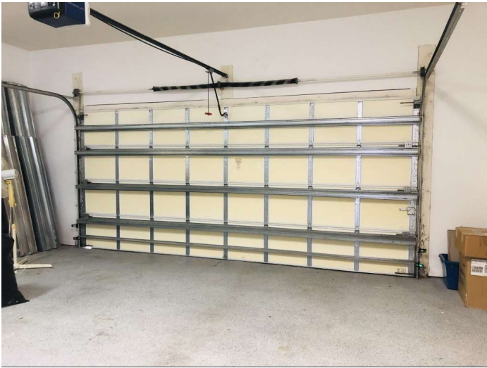
Non glazed wind resistant garage door with center beam support
