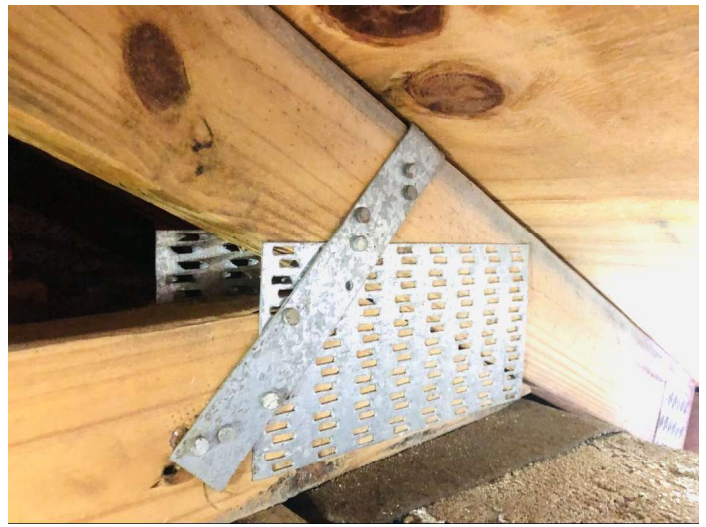
Single straps wrapped over trusses nailed per code
